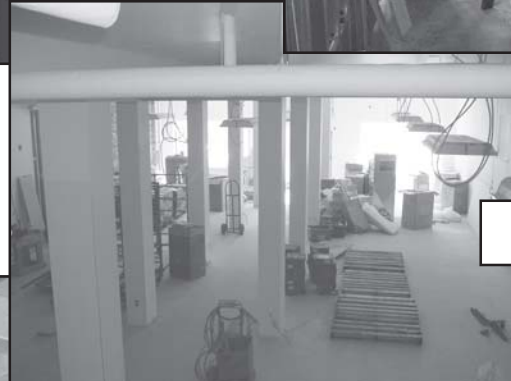
Apartments under construction at 66 Queen
